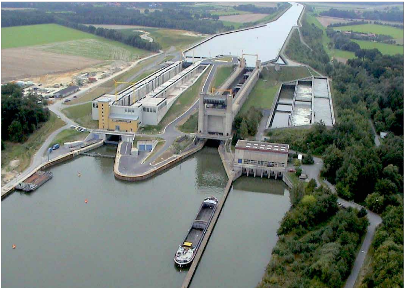
Fig. 3.3.1-1: Uelzen lock (Elbe Lateral Canal) [Waterways and Shipping Office Uelzen]
