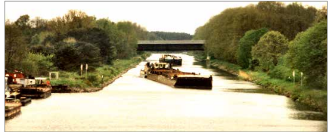
Fig. 4.1.7-1: Unladen ship sailing in strong wind (blowing from the right), which is relevant in the area with low trees [BAW]
